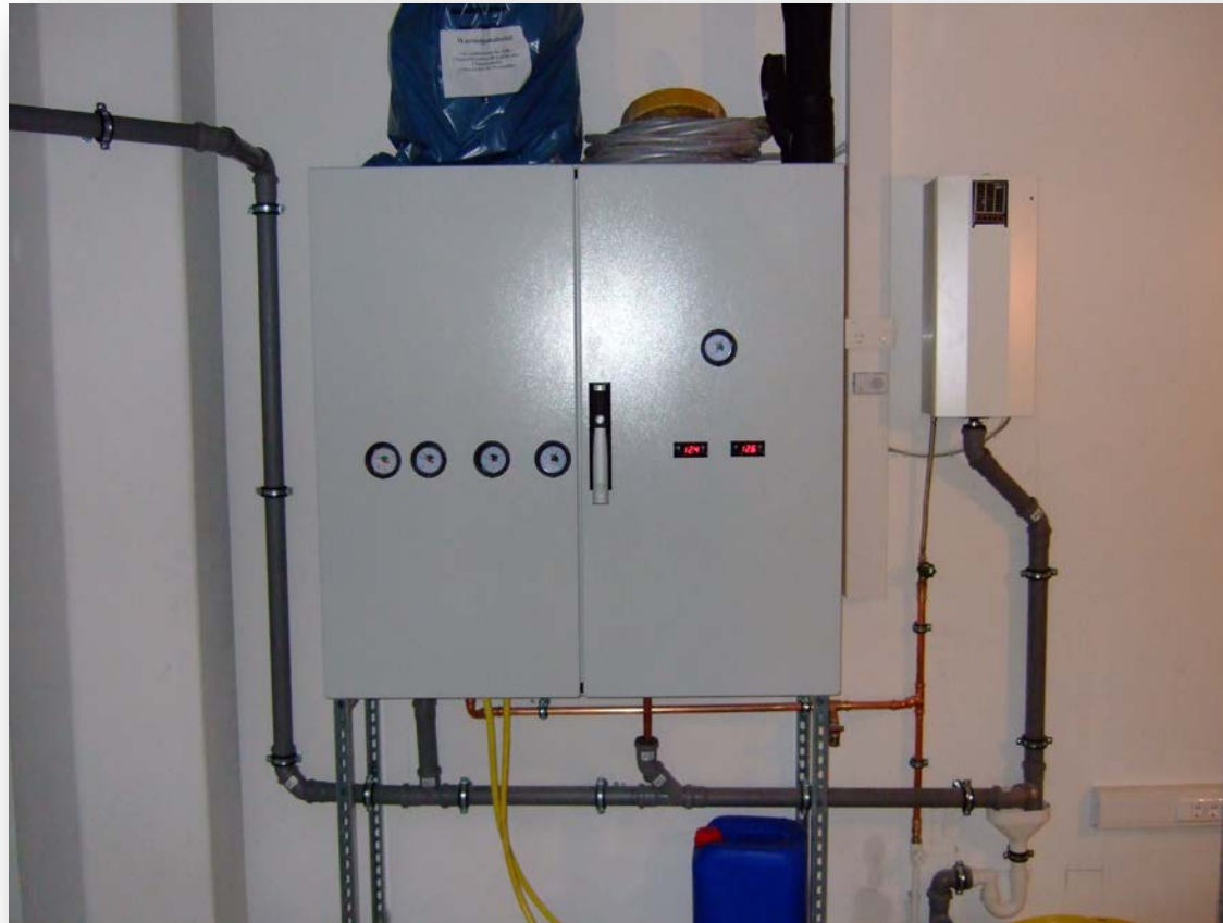
Water transfer station & Humidifier
